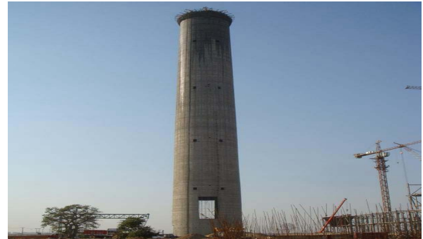
Jharsuguda IPP – 2400MW under construction
